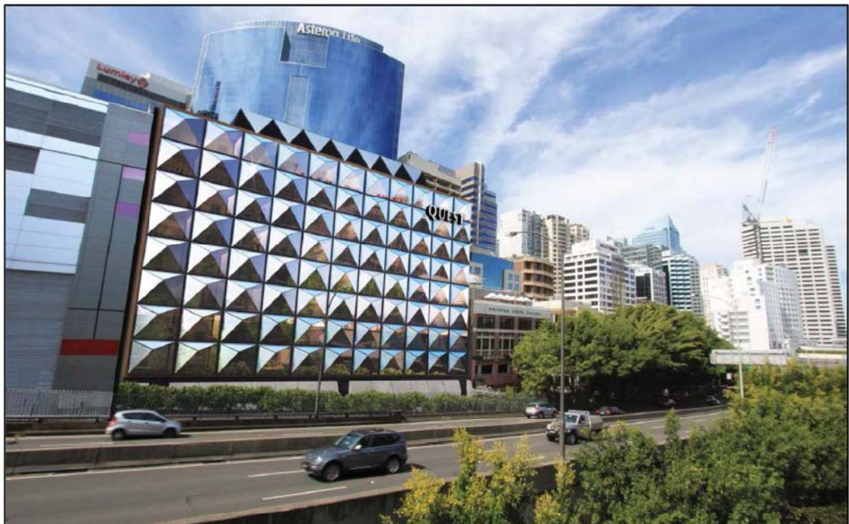
Figure 5 – Proposed development as viewed from west of the Western Distributor
